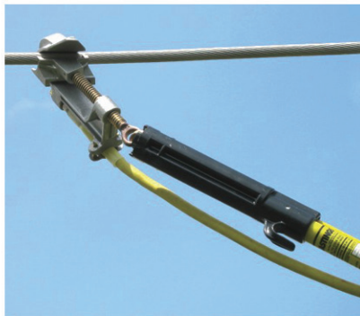
INSTALLING CLAMP
